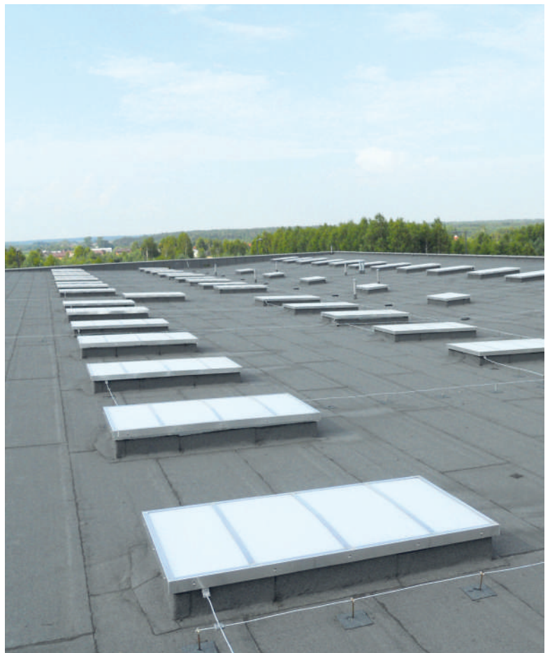
Fig. 10 – mcr PROLIGHT skylights
