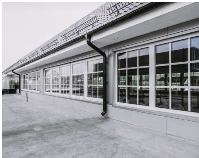
Fig. 35 – mcr OSO THERM smoke exhaust windows
