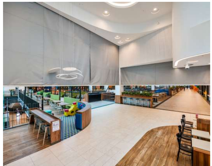
Fig. 44 – mcr PROSMOKE material smoke curtain
