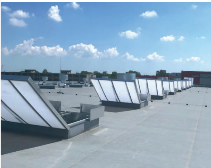
Fig. 7 – mcr PROLIGHT single leaf smoke vents, open
