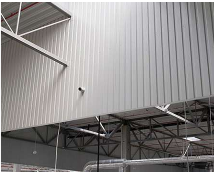
Fig. 43 – mcr PROSMOKE steel smoke curtain
