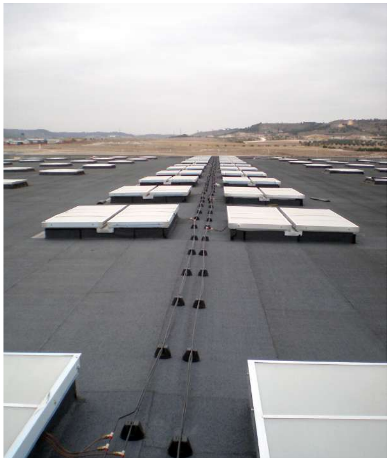
Fig. 6 – mcr PROLIGHT double leaf smoke vents
